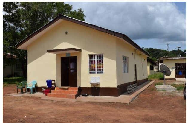
Vaccine storage facility at Kambia Government Hospital Credit: Tom Mooney, LSHTM
